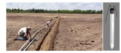
**Far left:** Installation of lysimeters at Byron Township site. Lysimeters are installed in holes at the bottom of the trench. PVC pipe protects plastic sampling lines from rodents.
